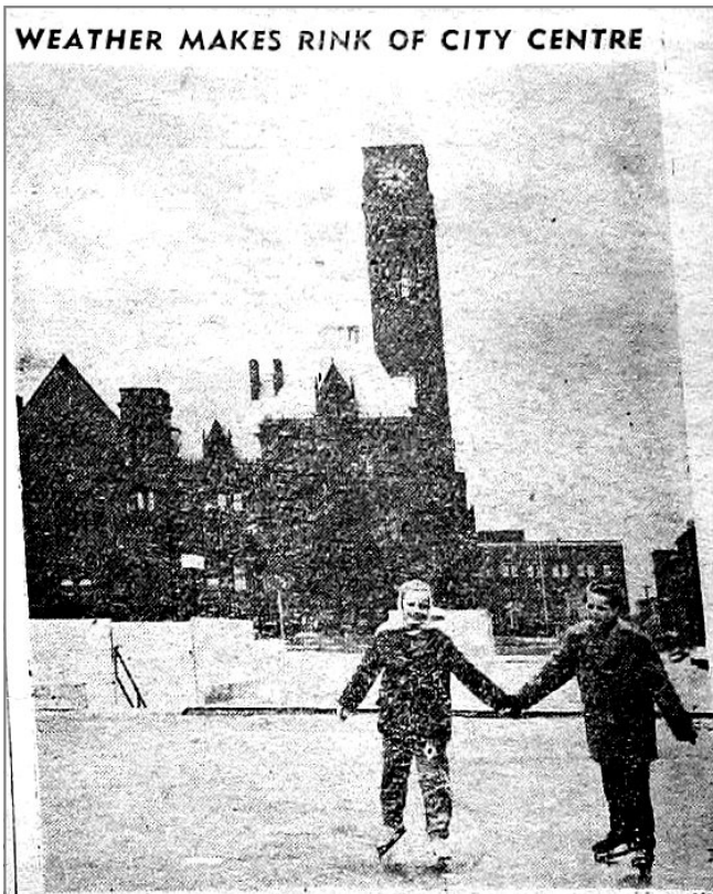
WEATHER MAKES RINK OF CITY CENTRE The underground parking garage at City Hall was built before the “new” City Hall. Freezing rain followed by a quick drop in temperature turned the top into “a perfect skating rink, probably the biggest in all Canada.” This was some years before the present rink was constructed.
